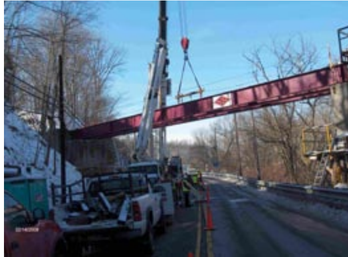
The final beam is set in place by Mingo Creek Construction
