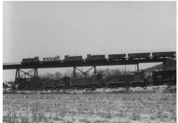
Empty hoppers cross McDonald Viaduct as a loaded coal train heads down the transfer track to deliver its cars to the interchange with the PRR Panhandle Division. Tim Sposato photo
