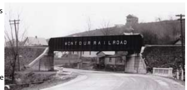
A 1930 view of the then new bridge over Route 30 in Imperial, which eliminated a grade crossing. County of Allegheny photo from Gene P. Schaeffer collection.
