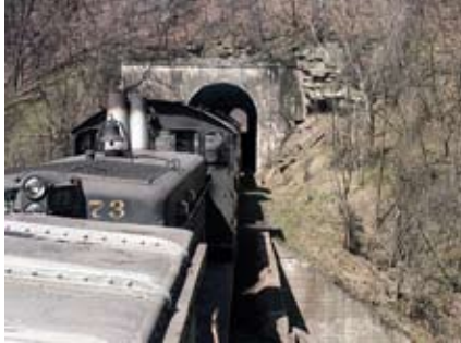
A view from a caboose shows a train crossing the concrete slab bridge before entering Enlow tunnel. A date stamp can be seen in the concrete bridge abutment. Roy E. Parkinson photo from Gene P. Schaeffer's collection.
