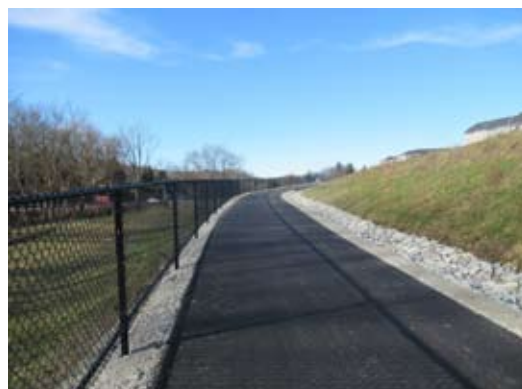
The asphalt paved ramp from the lower trail level looking west toward the Summit Drive Bridge. Photo taken 1/3/2022, after the safety fence was installed.
