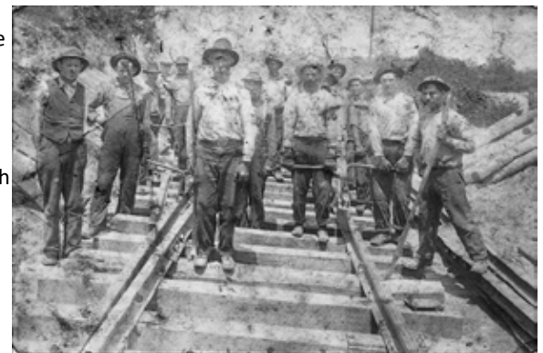
Track gang installs the east switch at North Star Junction near Imperial ca. 1913.
