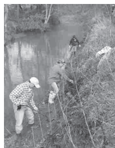
Left: Employees of Duquesne Light and Hazlett Tree Service of installing components of the branch-layered stream bank stabilization. Right - Branch-layered bundles awaiting bending over of stakes that will anchor them to the stream bank.
