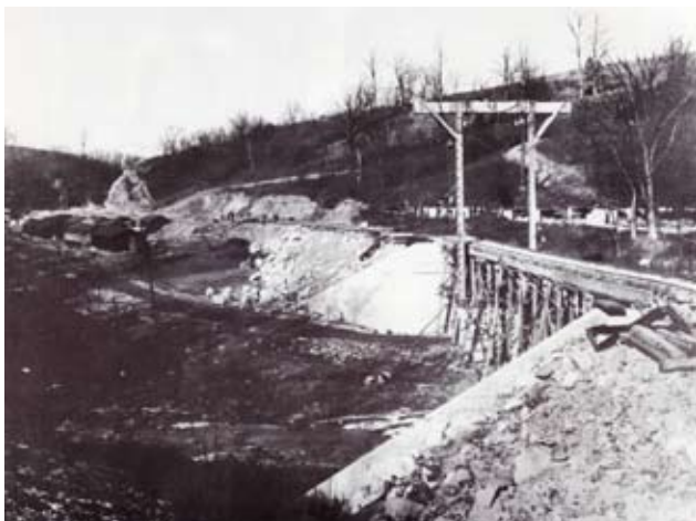
A construction camp is seen at the east end of Montour Mine #4 as the railroad crosses Valley Brook Road in Peters Township. This temporary wooden trestle was used during construction of the railroad until a steel plate girder bridge could be built. Photo courtesy Dave Richards / Gene P. Schaeffer collection.
