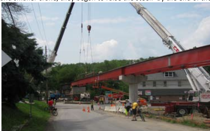
The first beam is set in place over PA 50 on the final day of steel erection. A Dennis Sims image.
