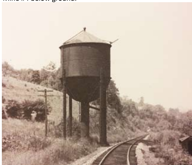
The steel Fife water tank sits beside the main line in the 1920's. Concrete footers for the four legs and the central column can be found near the edge of the trail. Photo from Gene P. Schaeffer Collection.
