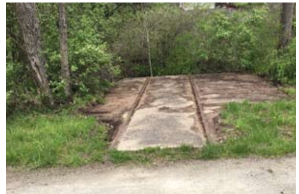
A concrete slab with rails embedded shows the former location of a tool house at trail mile 15. Bryan Seip photo.
