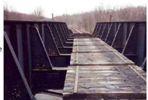
The U-shaped profile of a through plate girder bridge span is evident in this view of the Venice Bridge after abandonment of the railroad. Trains traveled between, or through, the main girders. Tim Sposato photo
