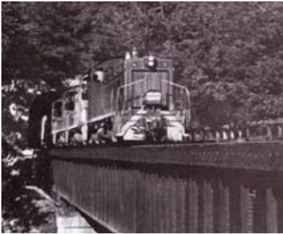
The bridge over Chartiers Creek is an example of a deck plate girder bridge. The large main girders are placed directly under the rails. Gene P. Schaeffer photo.
