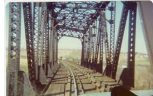
A view out the windshield of a track gang hi-rail truck as they transit the through-truss span of the McDonald Viaduct in 1976. The open framework supports a timber deck. Tim Sposato photo.
