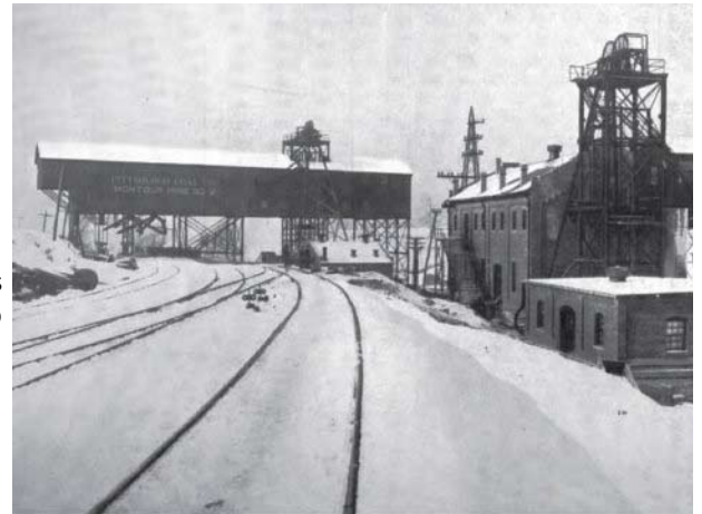
Montour #2 was a shaft mine, with support buildings next to the shaft in the foreground and the tippie building with its hoist shaft in the background. Photo courtesy Gene P. Schaeffer collection.
