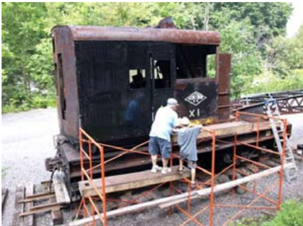
Bryan Seip and grandson work on the restoration of the X-1
