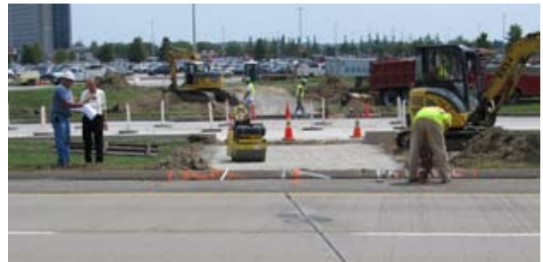
Contractor prepares sub-base and marks the curb where cuts will need to be made in the curb along the perimeter road on the west side of long term parking.
