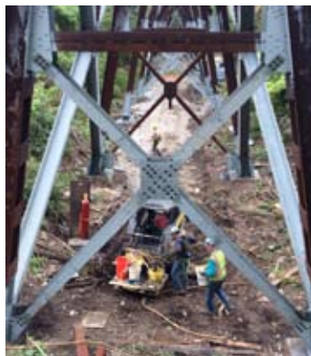
The photo shows some of the replaced steel (in gray).
