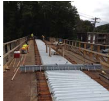
Photo shows some of the pans in place for the deck over spans 1 through 4.
