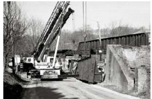
PennDOT removed two spans of the bridge in October 2001 to eliminate truck clearance restrictions. Gene P. Schaeffer photo
