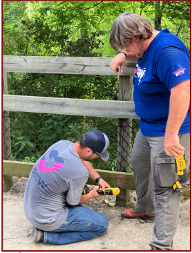
A fence improvement on the bridge in Venice.
