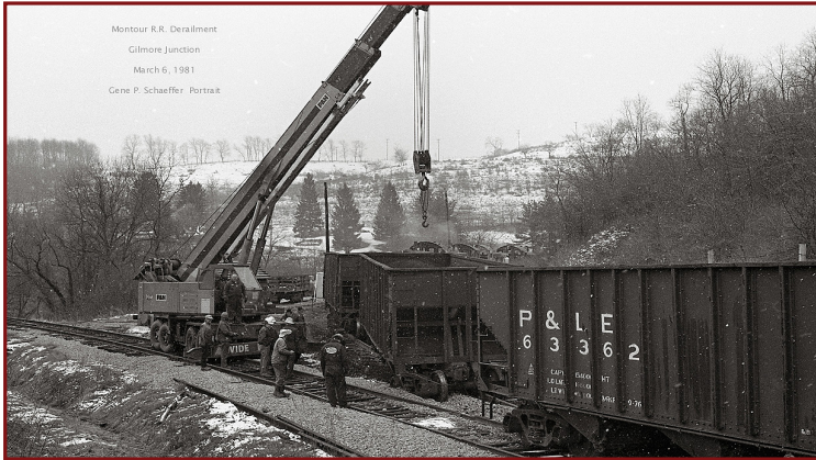
Empty hoppers headed to Westland derail at the Gilmore Junction switch, March 1981. A truck crane has been called in to rerail the cars. (photo: Gene P. Schaeffer)
