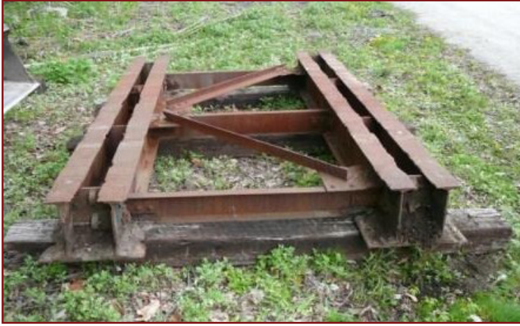
Lotus bridge relocated to Mile 30. The main I-beams and cross bracing are evident in this view without deck ties and rails.
