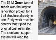
renovation project for a trail structure already in use. Early work revealed defects that tripled the original cost estimate. The steel arch support system will keep the 100+ year-old tunnel in service for the long term.
