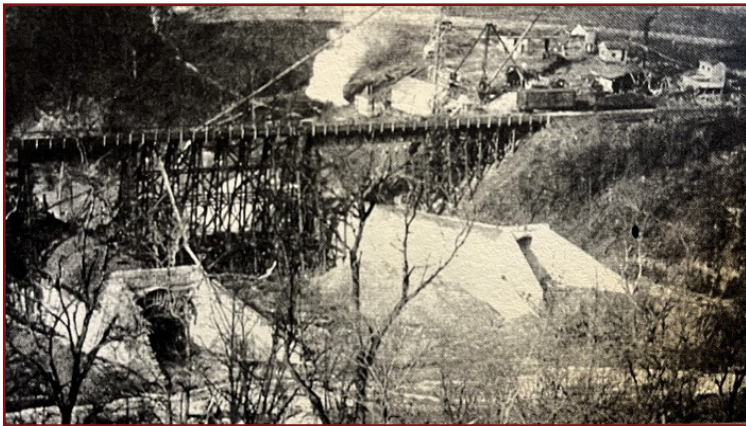
The tunnels under construction beneath the B&O trestle in 1924. (Photo: South Park Historical Society)
