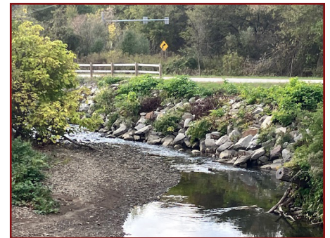
Past stream stabilization work
