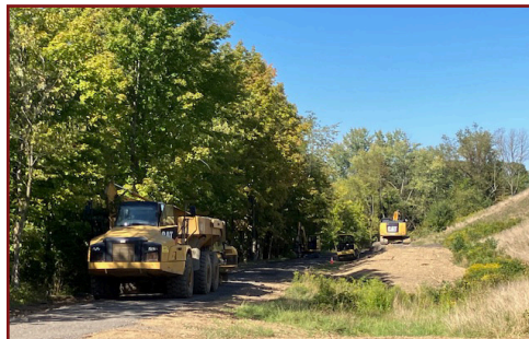
Muse branch under construction last summer.
