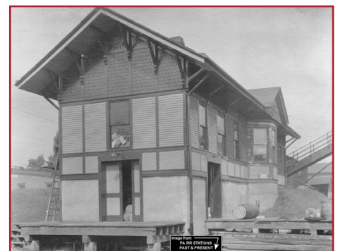
Rear view of the P&LE station. Note stairs on right side leading to an overhead walkway to the passenger platforms. (Photo: West2k.com)
