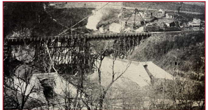
Construction of two tunnels under the B&O trestle in 1924. PRR Peters Creek (Green Man) Tunnel is on the right. (Photo: South Park Historical Society)
