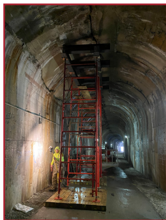
Shoring in the National Tunnel.
