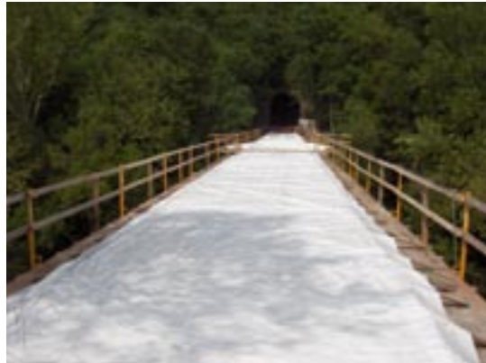
The deck for the Chartiers Creek Bridge was poured on Friday, July 11 lying in place as it cures. Photo by Troy Bogdan
