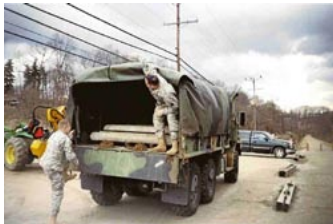
SGT William Shreve and SGT John Scheetz prepare to unload the concrete curbs near the Enlow Ball Field in Imperial.
