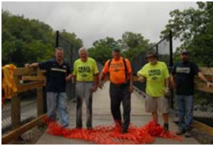
The construction crew pauses for picture; Tony Andrejasik (Beech), Bill Capp, Frank Ludwin, John Kozak (MTC volunteers) and Tom Crow (Trumbull)
