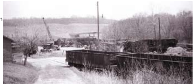
This 1956 view shows the yard at B&T. Two office buildings now occupy this site. Fred Bradley photo.
